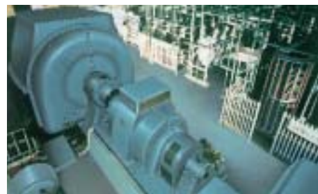
Short-circuit test generator No.1
