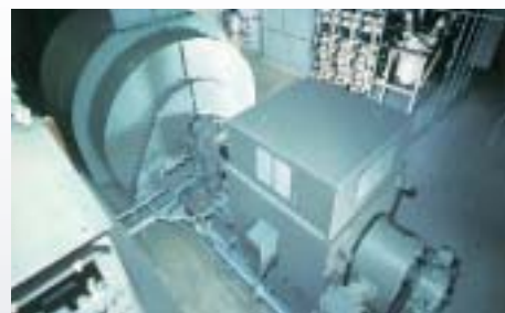
Short-circuit test generator No.2
